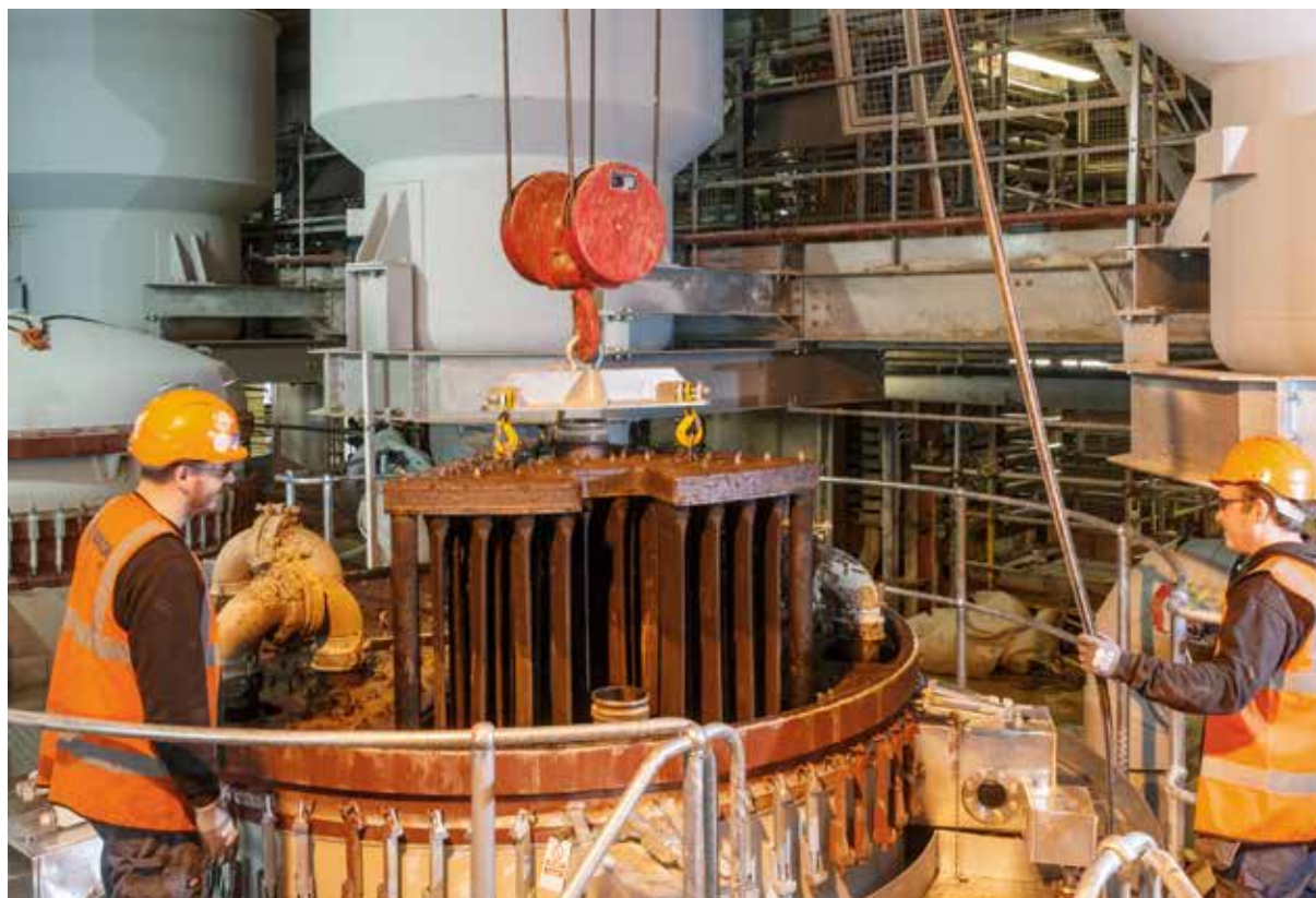
The filter vessel hold the filter segments with the mounted filter elements.
